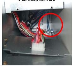
The cable from the adjacent dryer or home run will stay in this cavity.
